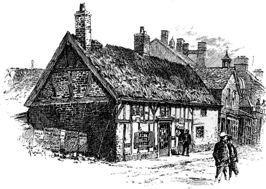
House gradually sinking.
